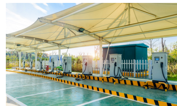
A combination of level 2 and 3 chargers provides challenging power quality issues which can be mitigated with proper transformer selections.
